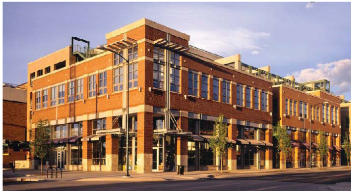
EXAMPLE Parking garage incorporated into overall building design.
