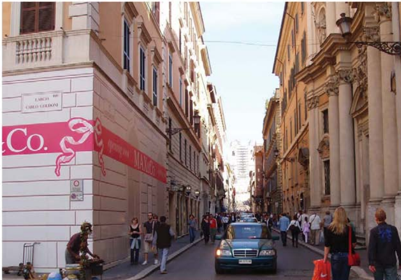
1.5:1 Street Wall Proportion, Via del Corso, Rome
