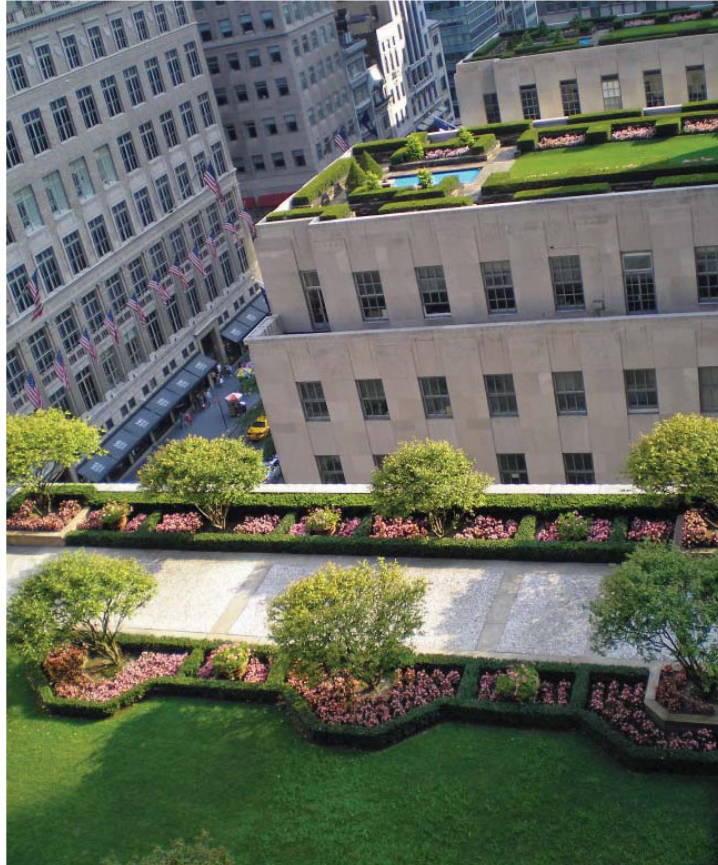
Roof of RCA Building, New York City
