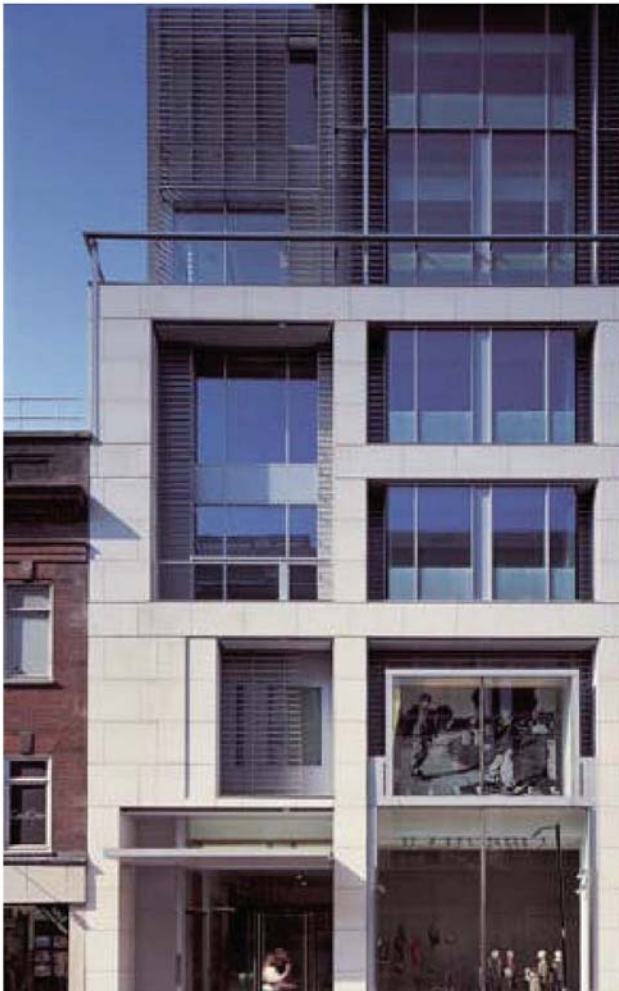
Lumina Building, London
